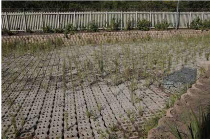
Figure 7: The newly constructed Bio-Swale with specially designed drainage system beneath and local vegetation for slow-treatment of runoff water. Slopes and grades are also designed to enhance sedimentation.
