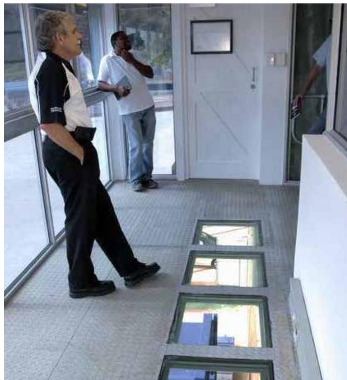
Figure 9: Illustration of the glass flooring so the Operator can see the compaction containers below and have full control of the system.
