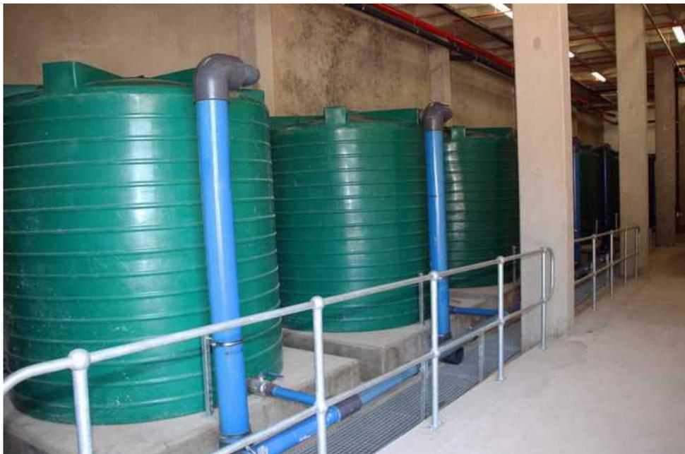
Figure 10: Rainwater tanks. This required special attention to sizing of tanks, piping, overflow, pressure and pumps. This water allows the Municipality to avoid using domestic water for non-consumptive usage (floor washing, vehicle washing, container washing, etc.)
