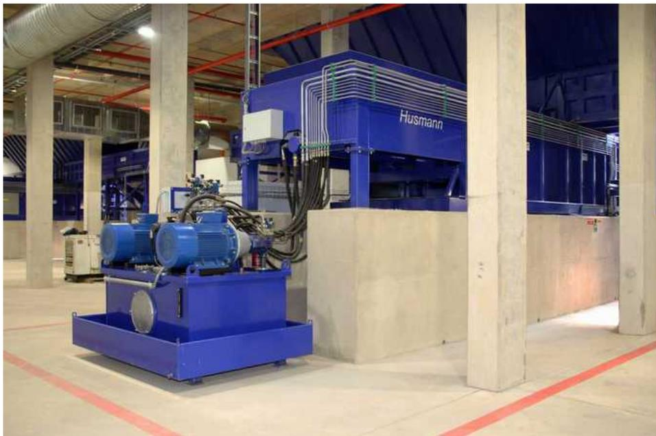
Figure 4: A main compactor ram unit which pushes waste into containers (containers are located outside the building). The compactor sits inside the building, on the floor beneath the offload platform (RTS floor).
