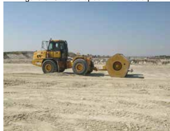
Figure 8: Compaction of cells
