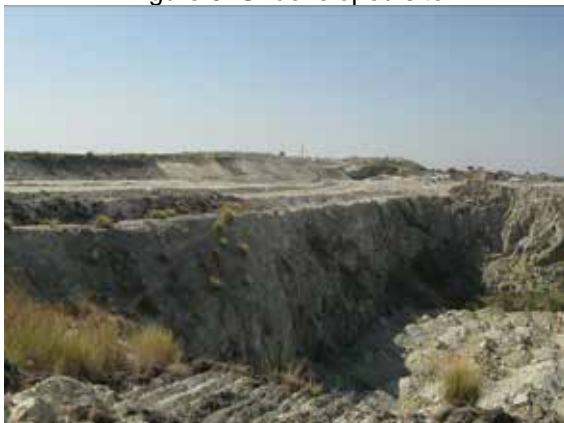
Figure 7: Rubble pit and cell construction
