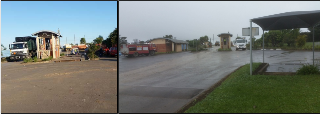
Figure 7: Repairs and Upgrades to the Weighbridge System
