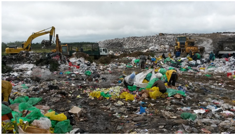
Figure 4: Uncontrolled Tipping of Waste outside the Lined Landfill Cell due to Inaccessibility to the Working Face due to Rainfall (No Wet Weather Cell Available)
