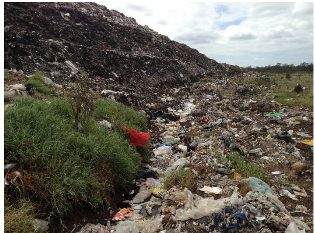
Figure 3: Steep Landfill Side Slopes due to Limited Lined Airspace
