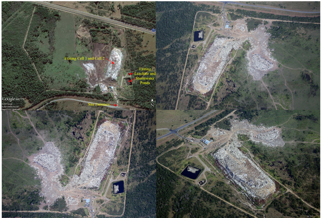
Figure 1: Aerial Photographs of the Roundhill Landfill Site
