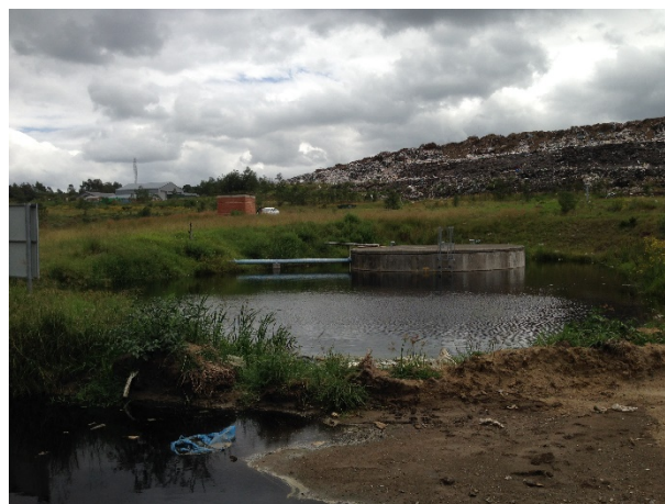
Figure 6: Uncontrolled Stormwater, Contaminated Stormwater and Leachate Runoff
